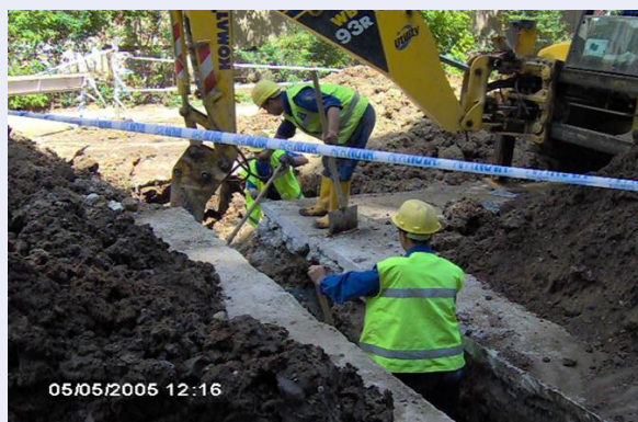
Water connection construction. (Photo courtesy of Apa Nova)
